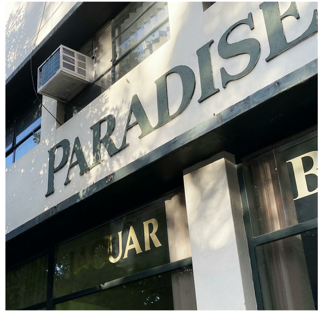
DARK GREEN OF EXISTING FACADE ELEMENTS CONSERVED AND REPAIRED
